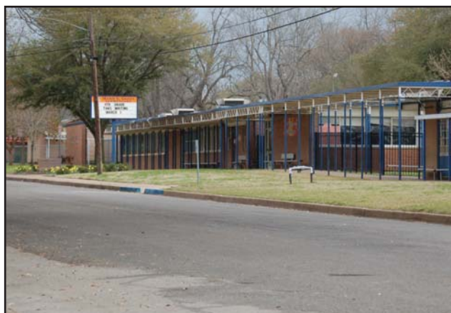
Old Griffin Elementary site
