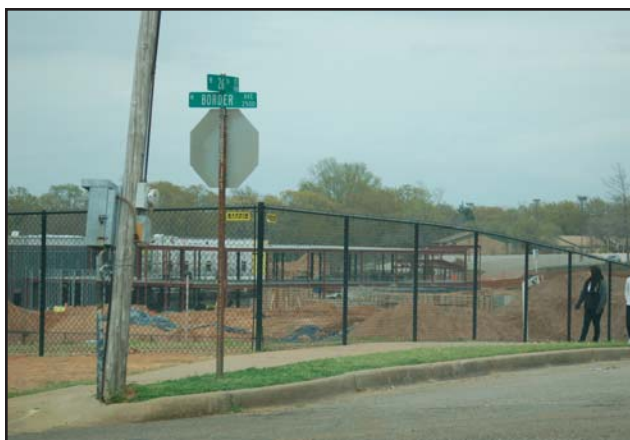
Construction of the new Griffin Elementary School
